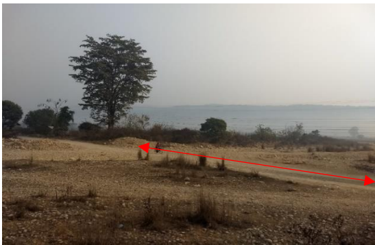
Fig11.3: D/S of Andheri Khola from u/s right side with marked bridge axis
